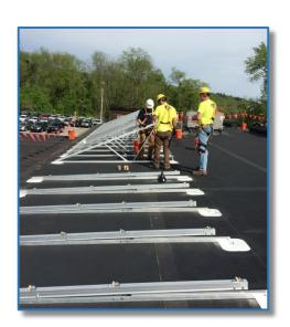
The new solar system will be used as a training tool for apprentices as well as other members of the local. Specifically, the system will include 64 solar panels with micro-inverters, all components being American-made. The estimated annual production of the system is expected to be 17,800 kWh, which will satisfy over 60% of the building's electrical needs.
